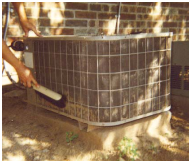
Keep your unit clear of high grass so that it can pull in plenty of fresh air. Coil blockage increases operating cost and shortens equipment life cycle.
