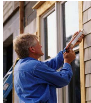
A little time spent with a caulk gun and scraper can save energy and prevent costly repairs from water damage. Take a look at your windows, doors and plumbing penetrations and make sure they are sealed.
