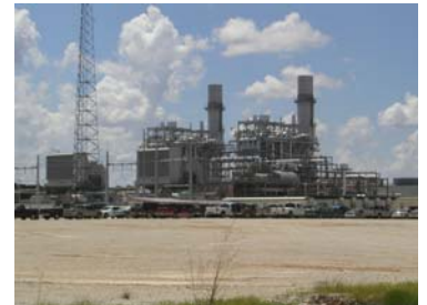
This Jack County Combined Cycle Power Plant operated by Brazos Electric Power Cooperative helps to meet your Cooperatives demand for energy. New power plants will be needed in the future to meet the demand for electricity.
