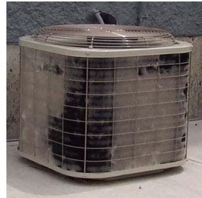
Dirty coils increase operating cost and can cause serious equipment failure. Keep them clean and save!
