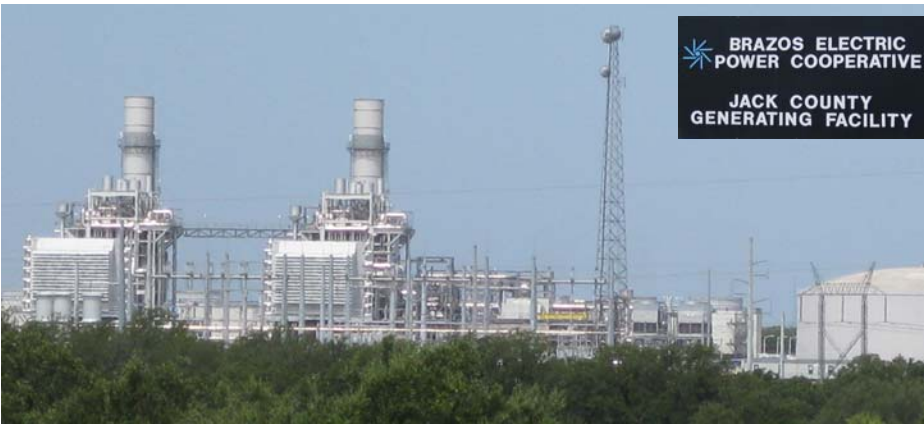
The above picture is of the 620 MW Jack County generating station unit 1. A second station similar to unit one is under construction at this time and scheduled for completion in the second quarter of 2011. Unit 2 will be located on the same property and double the output of electricity. Planning for the future power needs of our members is critical for maintaining power quality.
